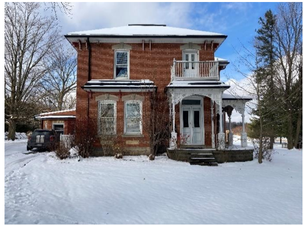
Plate 8: Farmhouse at 1420 Charleston Sideroad
