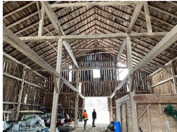
Plate 40: Interior frame structure of the barn
