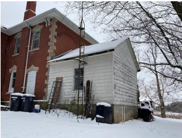
Plate 35: East and south elevations of rear addition
