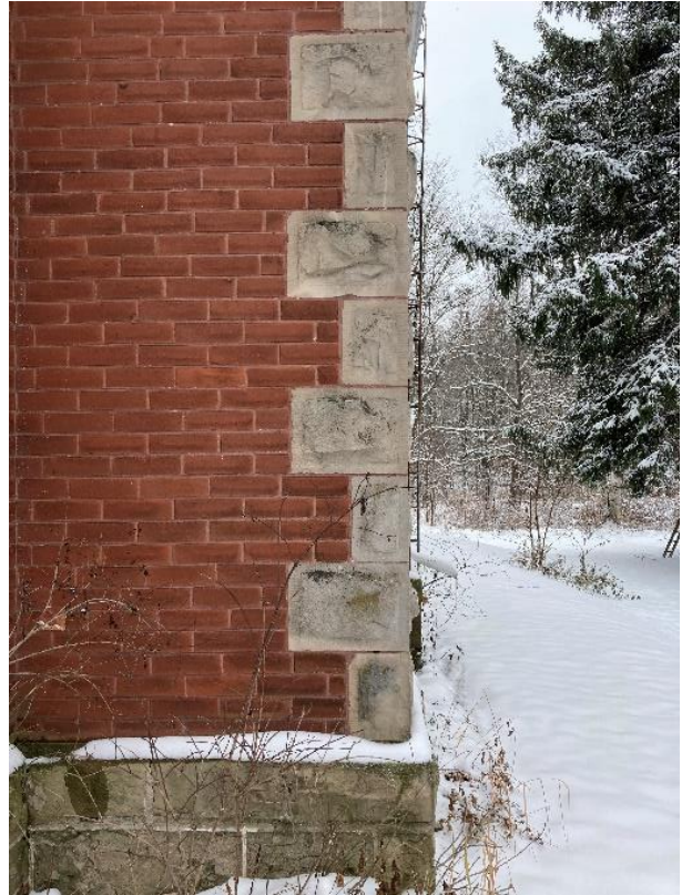
Plate 22: Representative example of stone quoins
