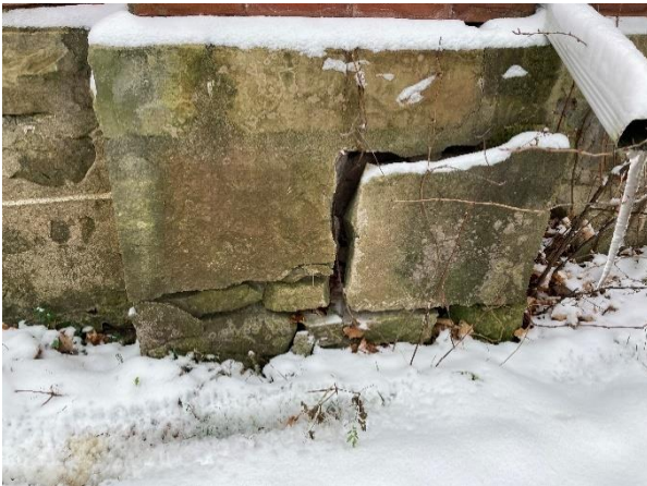
Plate 27: Deterioration in the foundation of the west chimney on the west elevation
