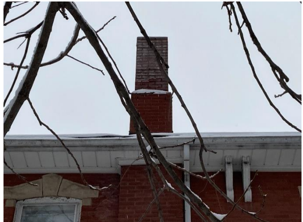
Plate 28: West chimney of west elevation
