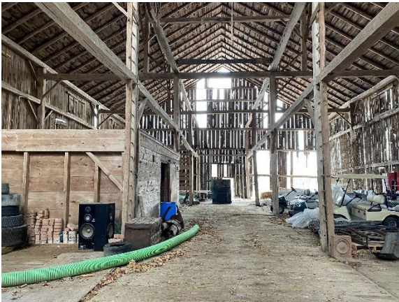
Plate 39: Interior frame structure of the barn
